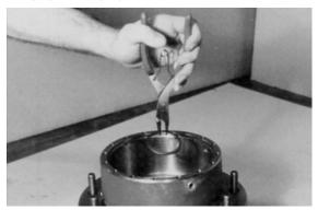
11. At this point the hub-spindle sub-assembly is complete.
